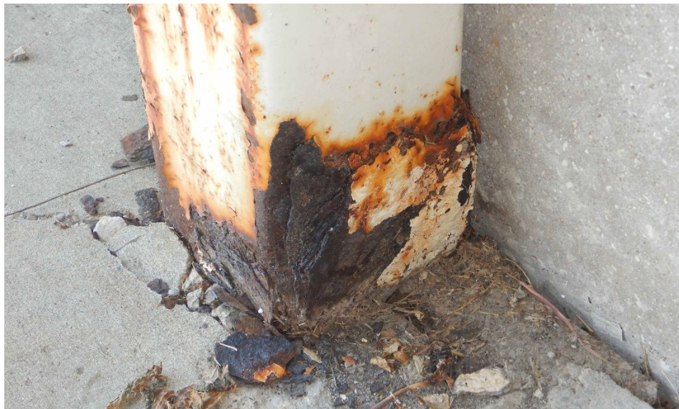
Photo 10 – Deteriorating structural steel column at covered parking – west side of building.
