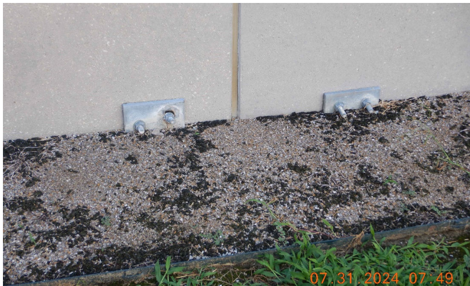
Photo 9 – Field modified base connection
