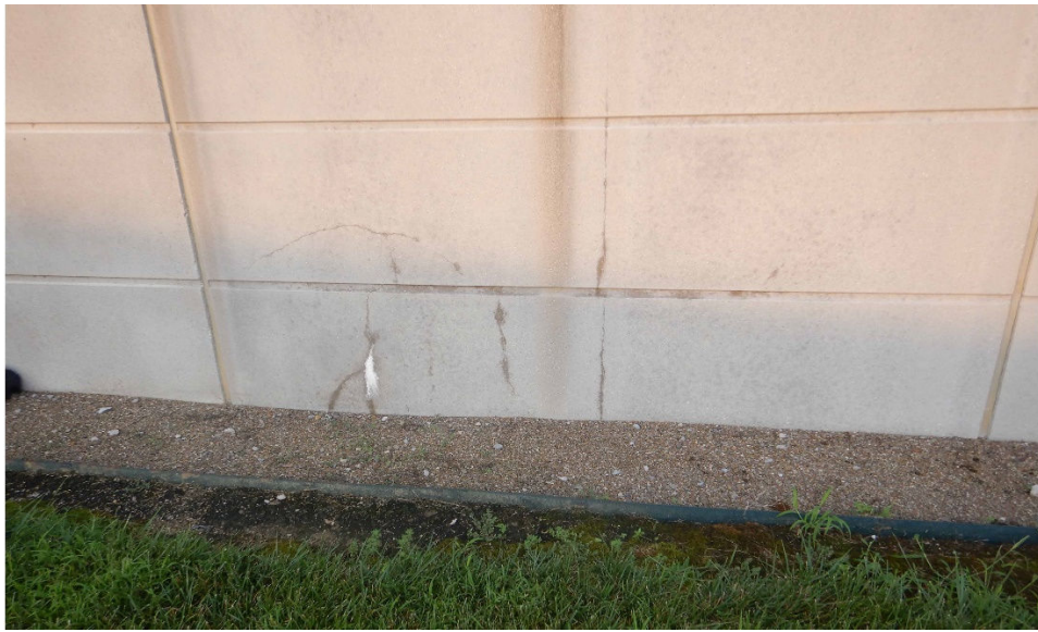
Photo 5 – Shrinkage cracking in face of pre-insulated precast concrete panel.
