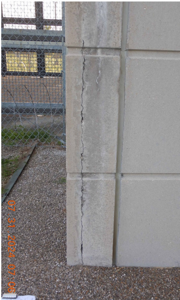
Photo 1 – Exposed-to-view end of pre-insulated precast concrete wall panel. Vertical crack typical.
