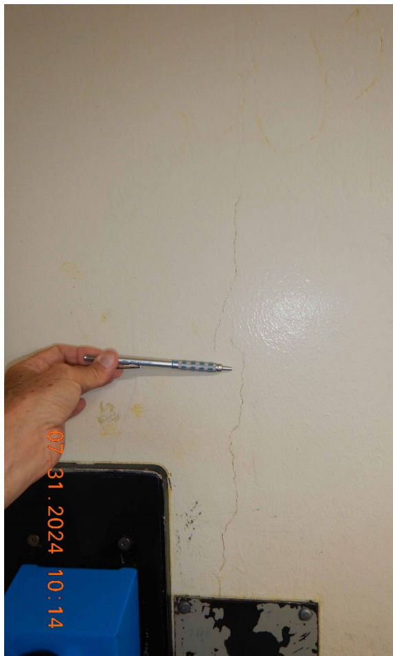
Photo 11 – Vertical crack that is commonly found in the vicinity of the phones in the detention cells
