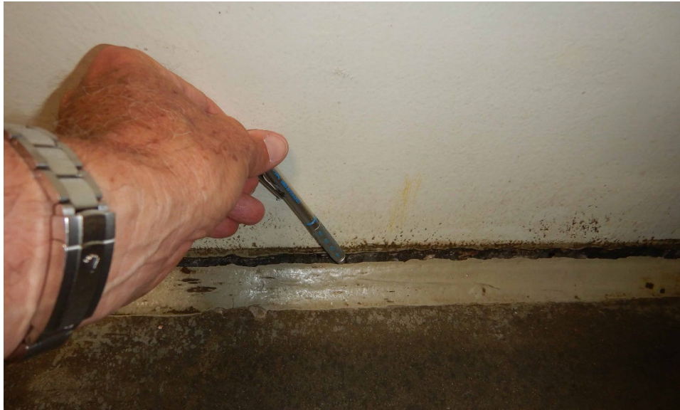
Photo 15 – Separation between exterior precast concrete wall panel and mezzanine level floor.
