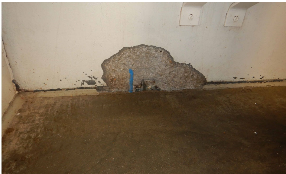
Photo 12 – Duct and embedded Unistrut that is common just below phones in cells
