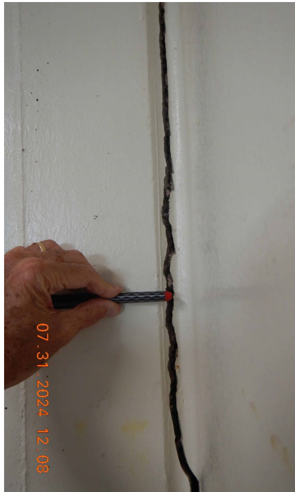
Photo 14 – Vertical separation between exterior precast concrete panel and interior precast concrete column
