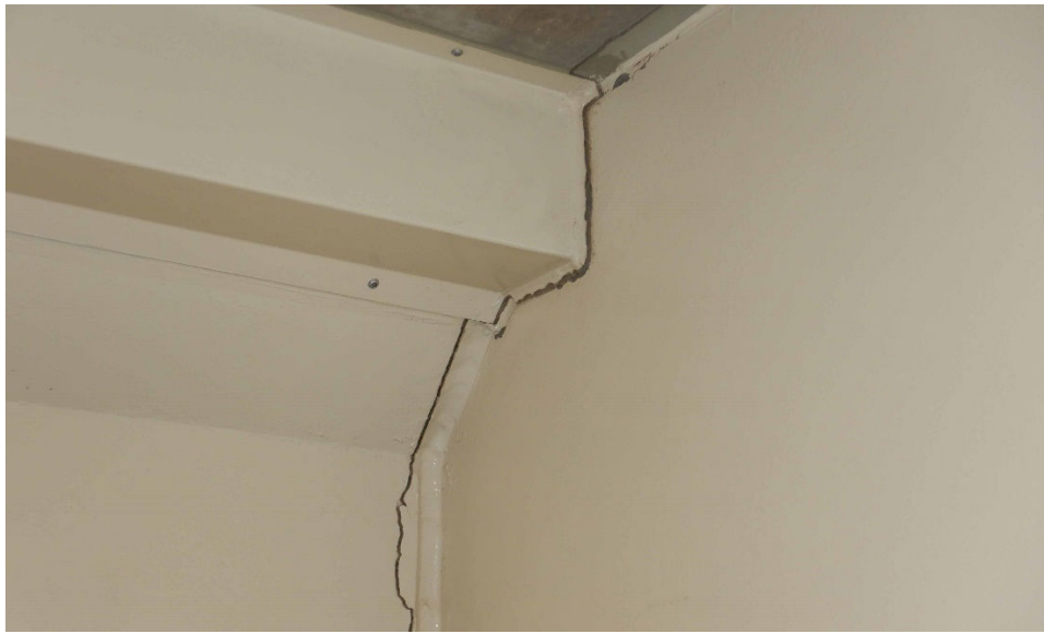
Photo 17 – Separation between precast concrete wall panels at building corner.
